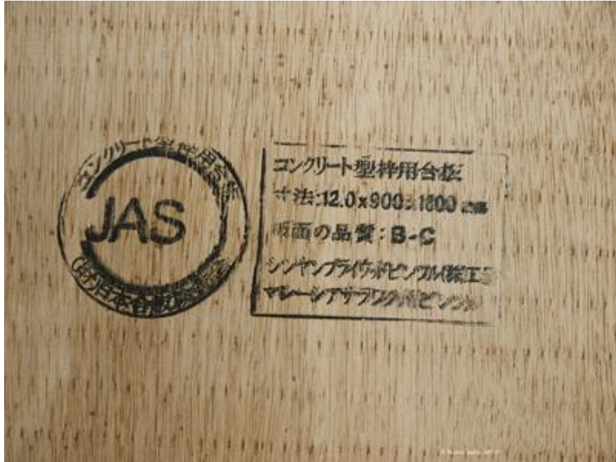
JAS Concrete Form Plywood 12mm
